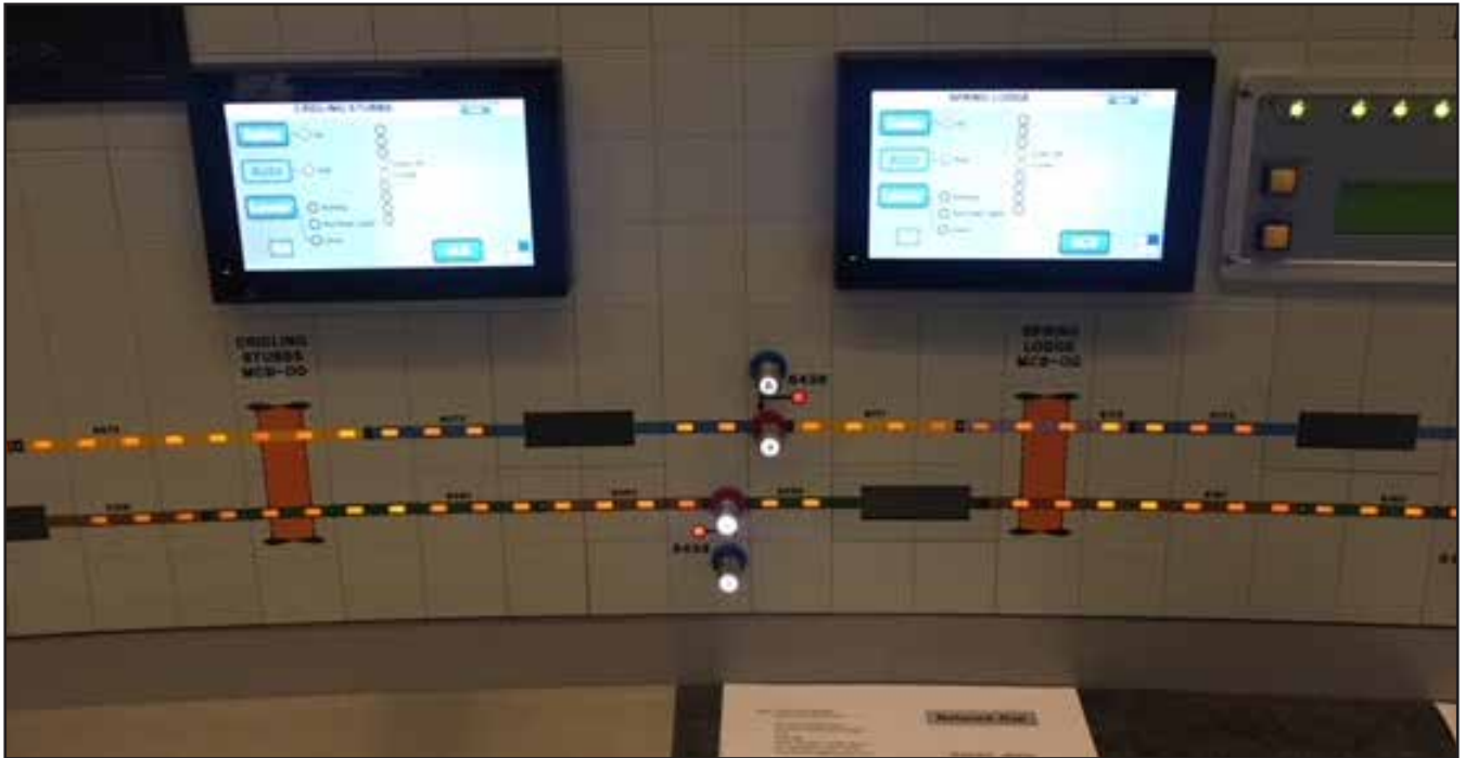
© Network Rail, Ferrybridge Signal Centre
